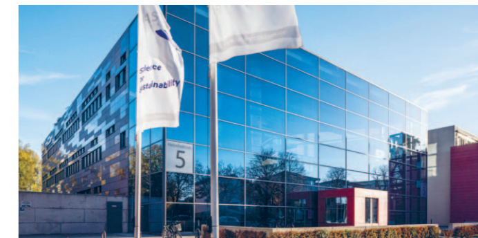
The office building on Helmholtzstrasse. © Rolf Schulten
