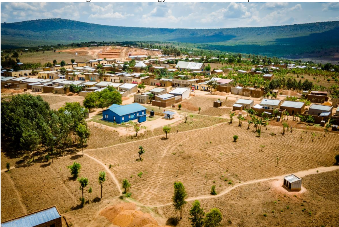
Local networks provide solar energy in this settlement in the Eastern Rwandan district of Nyagatare. TU BERLIN/Pacifique HIMBAZA
