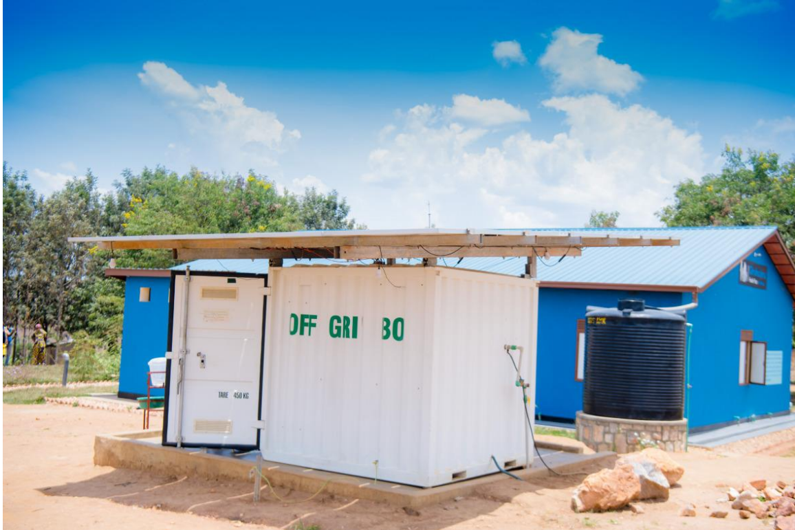
Off-grid boxes equipped with solar panels and a water purification system. TU BERLIN/Pacifique HIMBAZA
