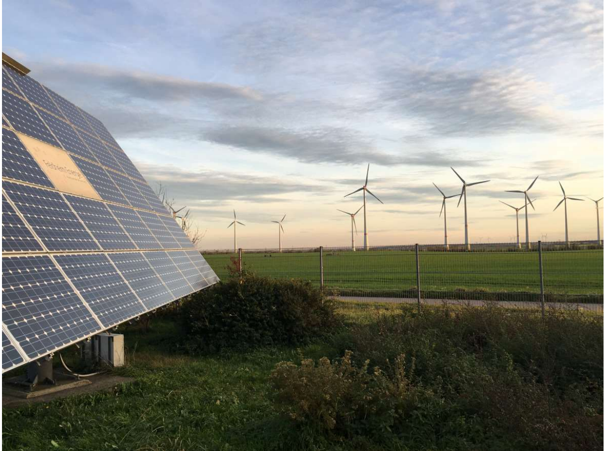
This self-aligning photovoltaic module follows the movement of the sun to optimize efficiency. IASS/ S. Letz
