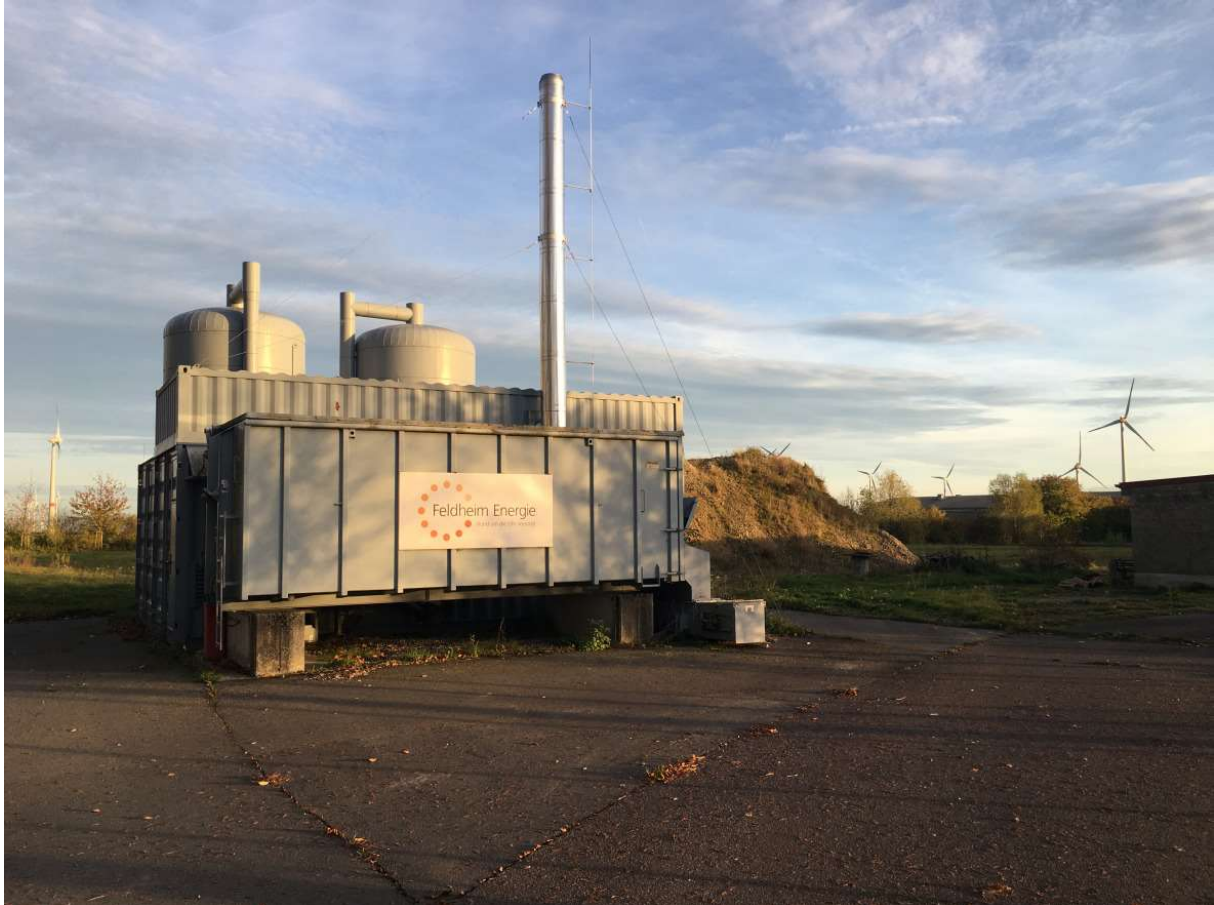
This biogas plant is fed with pig and cattle manure as well as corn silage and grain meal from local farms. IASS/ S. Letz
