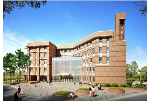
Figure 5: ICTC building, Pulchowk campus (Project site)
